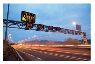
Regional control rooms oversee the motorways, but much of the traffic management is carried out automatically. automatically. For example, sensors in the road detect how fast traffic is moving, and therefore whether a queue is beginning to form. If this happens, they can send a message to overhead gantries or roadside signs warning drivers of congestion ahead and setting appropriate speed limits.
